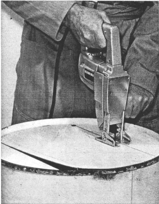
Ash-dumping doors fit into a 10-in.-wide opening sawed out of the bottom of the 30-gal. drum. Orient the cutout so drum seam will be at rear of burner
