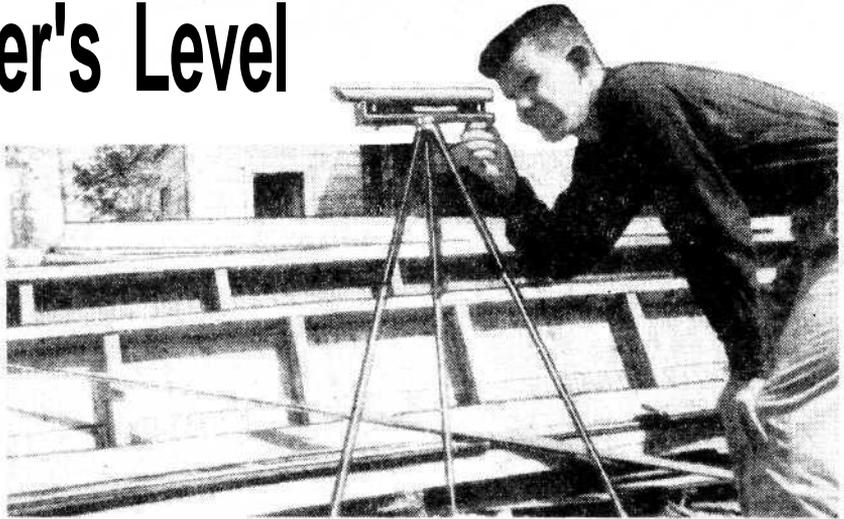
**1** Using engineer's level on a camera tripod to set concrete forms.
