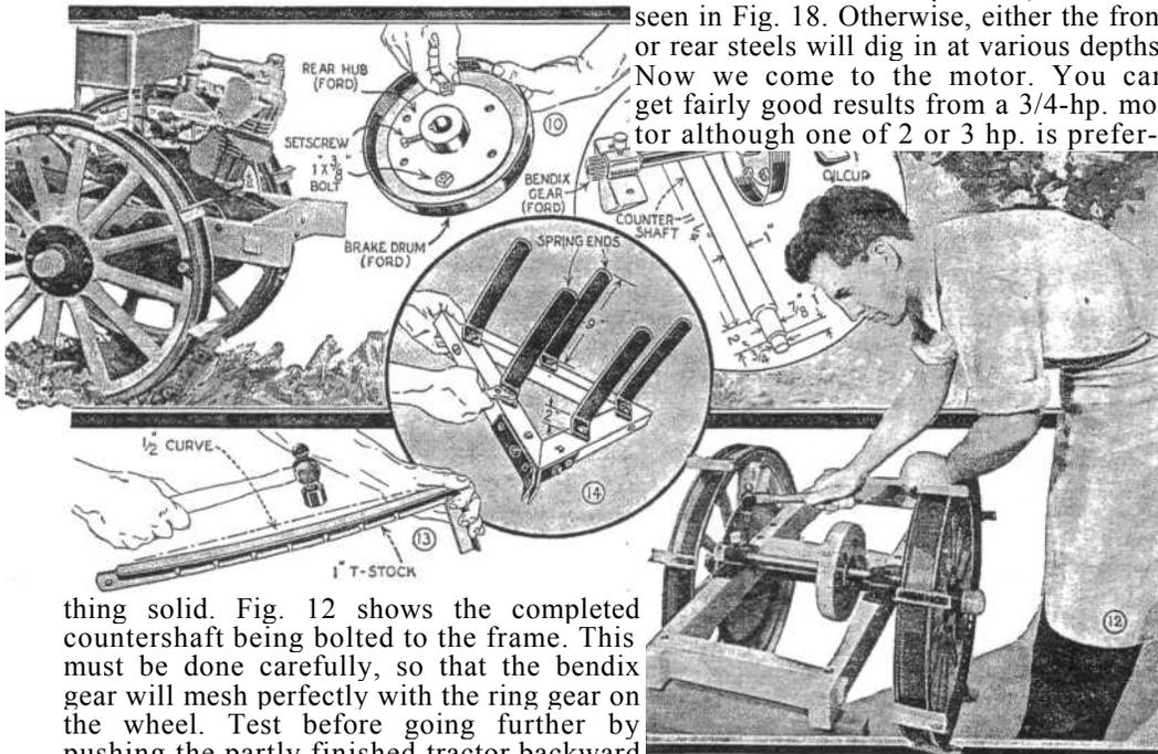
thing solid. Fig. 12 shows the completed countershaft being bolted to the frame. This must be done carefully, so that the bendix gear will mesh perfectly with the ring gear on the wheel. Test before going further by pushing the partly finished tractor backward and forward across the floor.
