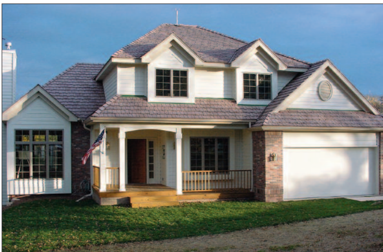
Build A Better Home research demonstration house USDA Forest Products Laboratory; Madison, Wisconsin
